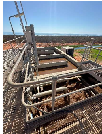
Plate 4: Wastewater Treatment Plant – Biological Reaction Process with Ultrafiltration Membrane System
