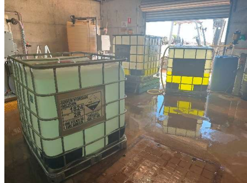
Plate 8: Wastewater Treatment Plant (sodium Hydroxide Intermediate Bulk Container (IBC))
